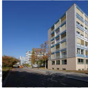
2 Faculty of Mechanical Engineering and Faculty of Electrical Engineering, CTU (F. Čermák, G. Paul, J. Liberský, V. Hladík, 1958–1969; restored)
