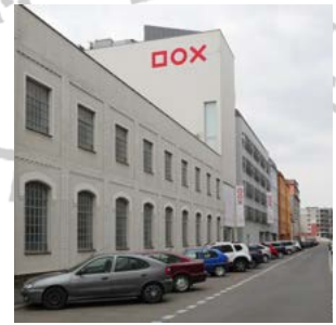
12 DOX – Centre of Contemporary Art / Rossemann & Kühnemann Mechanical Engineering Factory (A. Žižka, F. Troniček, 1901, 1928–1930; I. Kroupa architekti, 2007–2011, radical adaptation)
