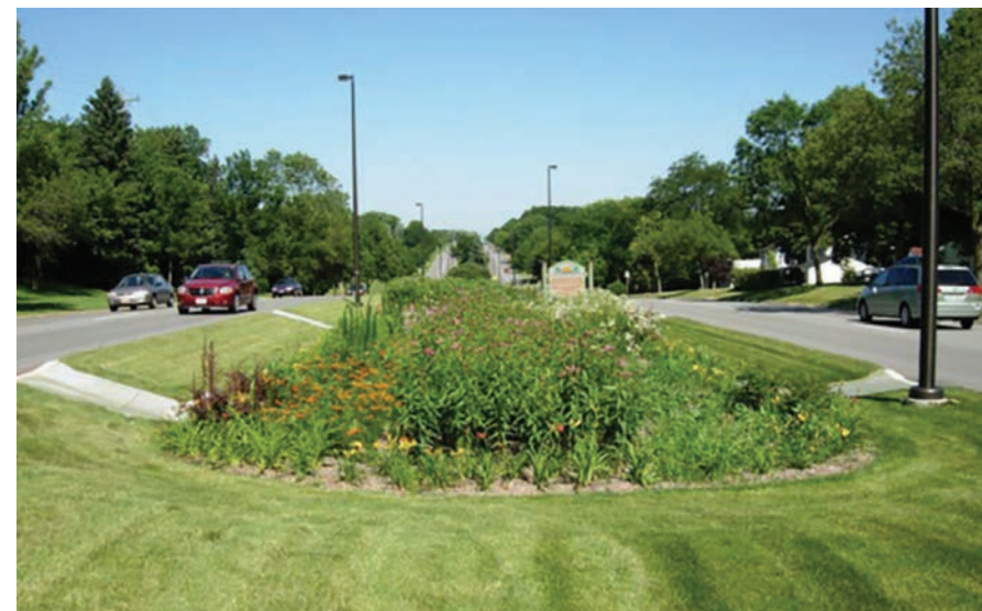
Fig. 2. Dry-swale a High Point, Seattle, Washington 2010 (fonte: Brett VA, via Wikimedia Commons).
